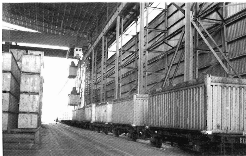
Container handling and storage under cover.
